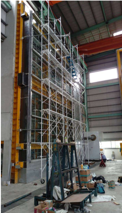
Completed Installation of Curtain Wall Corner at CT-370CB
