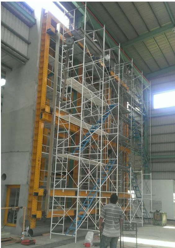
Installation of Curtain Wall Specimen at CT-
