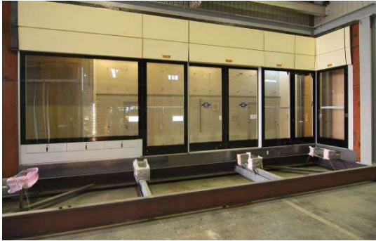
Installation of Prototype Platform Screen Door
