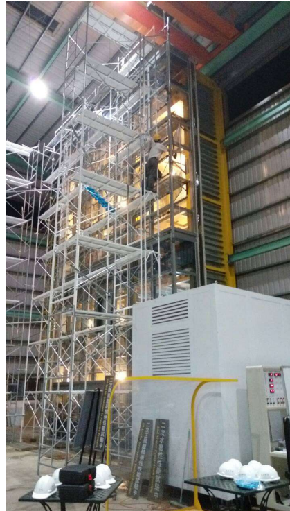
Dynamic Water Penetration Test for Curtain Wall Corner at CT-370CB
