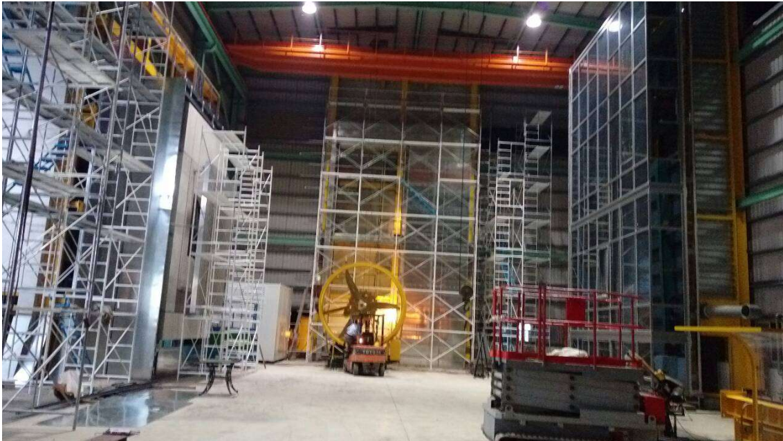
Installation in Progress at Chamber CT-310C
